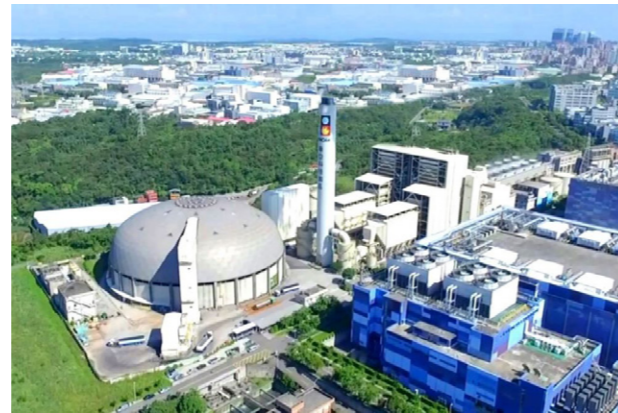
EPC Integration Services For Power Generation
