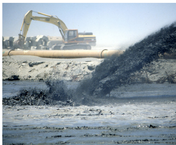
Pumping sand to fill the sea
