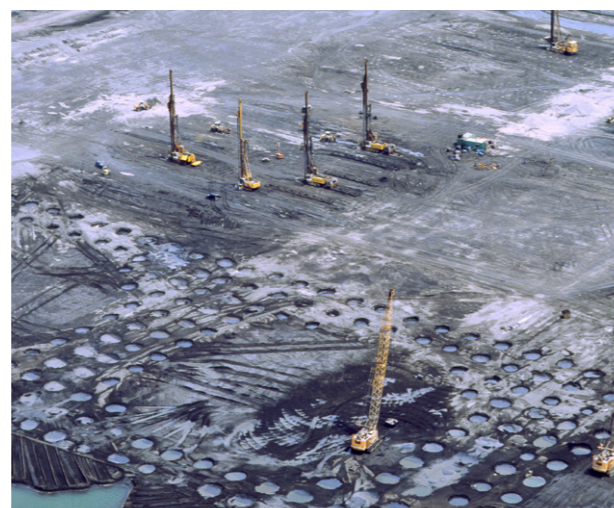
Around the clock ground improvement to consolidate the foundation
